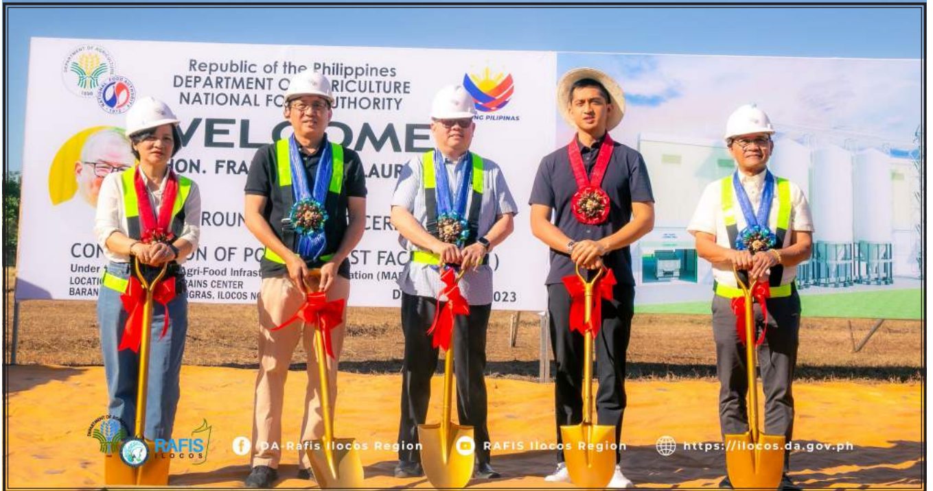
Agriculture Secretary Francisco Tiu Laurel, Jr. and Ilocos Norte Governor Matthew Marcos Manotoc led the groundbreaking rites for four units of large rice dryers in Dingras, Ilocos Norte. To be constructed under the National Food Authority (NFA), the drying facility will enhance the agency's procurement capability, increase rice yield, and boost rice and corn storage capacity. Valued at P130 million, the project will be built in 10 months, in time for the main rice harvest season in 2024. (Photo courtesy of DA I – RAFIS)
