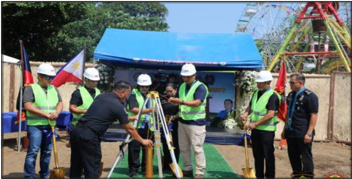
Bureau of Fire Protection Regional Director CSupt Leonida Rosales, together with BFP R1 Command Group, and Pagudpud municipal officials headed by Mayor Raffy Benemerito II, led the groundbreaking ceremony for the construction of a new fire station project in Pagudpud, Ilocos Norte. The ceremony was held on April 27, 2023. (Photo by BFP-PIU/Ilocos Norte)
